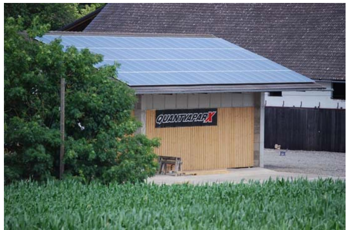
Solar panels to charge batteries
